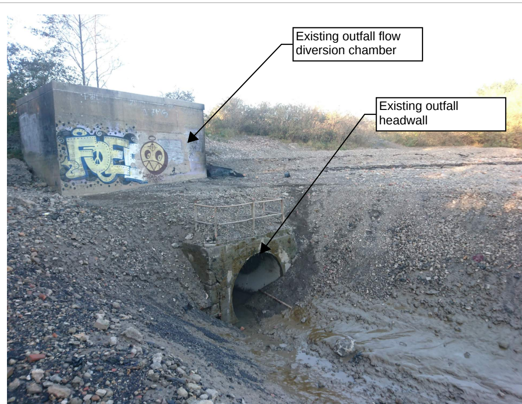
Existing outfall headwall Photo
