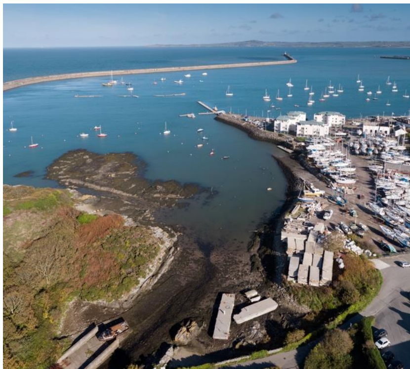
Figure 20. Aerial image of Porth y Felin. The river runs across the shore in the foreground past the remains of three floating breakwater pontoons. The recovered wreckage is on the hard standing on the right. Photo. R. Holt.
