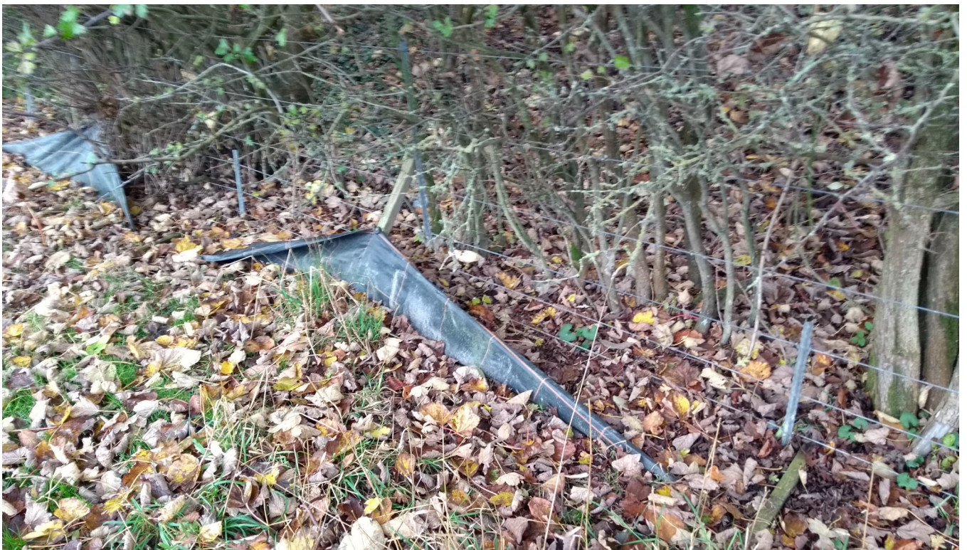
Image 6: Geotextile supported by wooden poles. Facing south.
