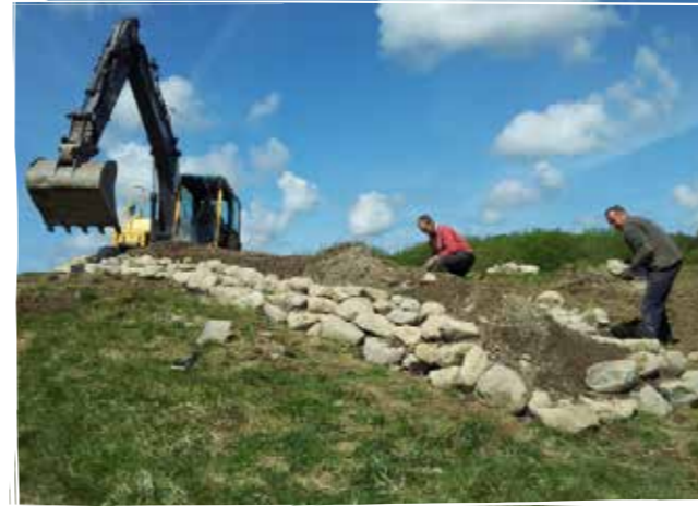
Finishing off with local boulders
