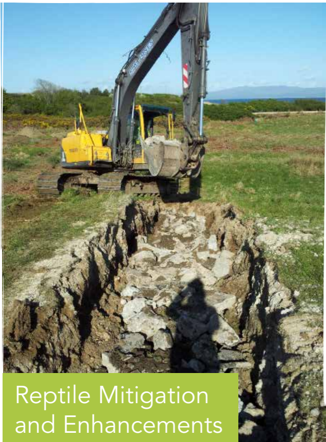
Excavation of deep trench and infill with rubble
