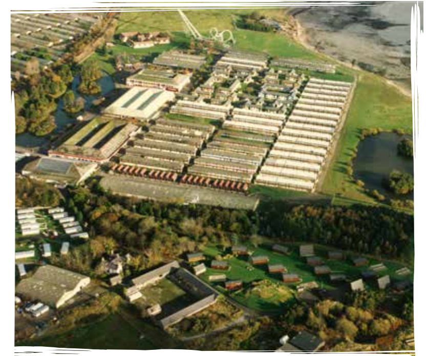
The southern part of Starcoast World - extensive chalets and Boomerang rollercoaster - that was visually intrusive. Chalets required significant investment to create Hafan y Môr
