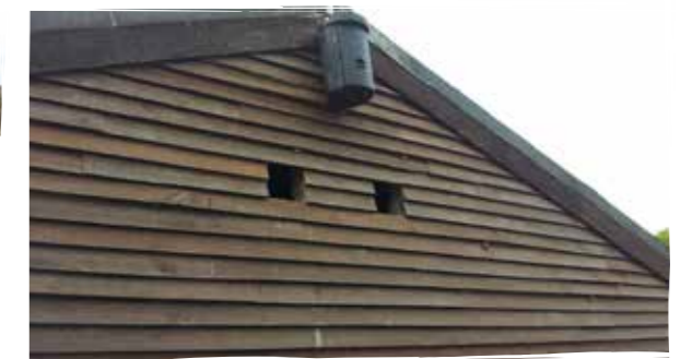
Old chalet retained and converted to provide bat roosting facilities
