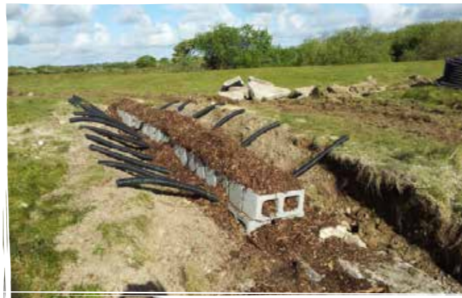
Installation of chambered blocks with bark fill as hibernation sites and reptile access 'tunnels'
