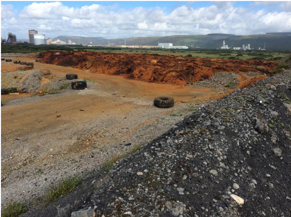
Plate 6-1 View North over MNHL Cell 2. Note dominance of iron rich filter cake
