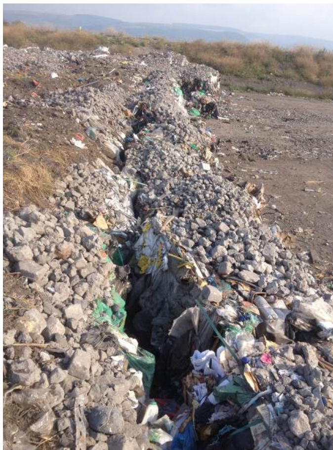
Plate 4-1 Gaps between bales in bio cell
