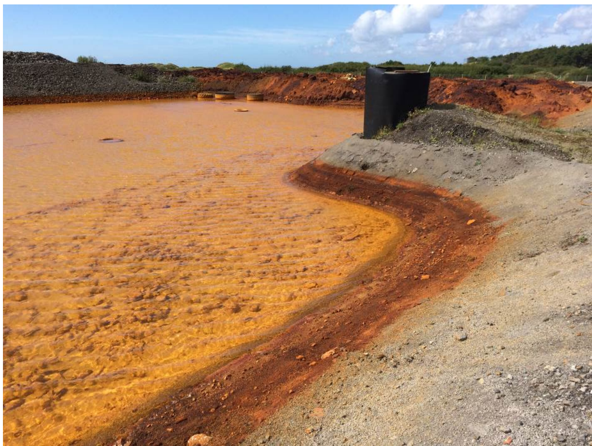
Plate 8-1 Cell 2 leachate sump L8. Note staining due to iron.
