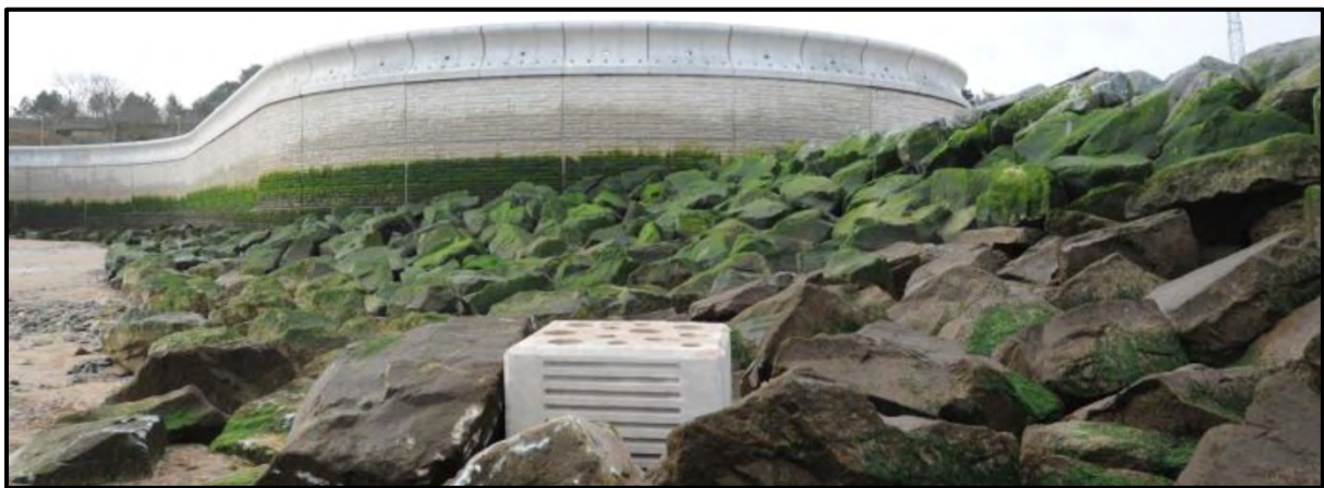
Image 18. Bioblock positioned within rock armouring at Colwyn Bay
