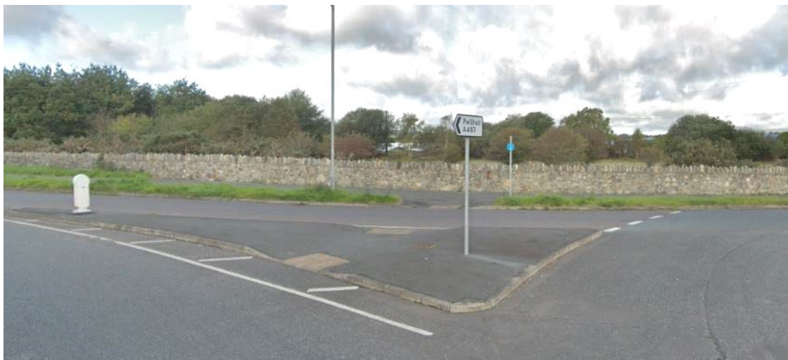
Figure 3-3: Crossing points on Links Road
