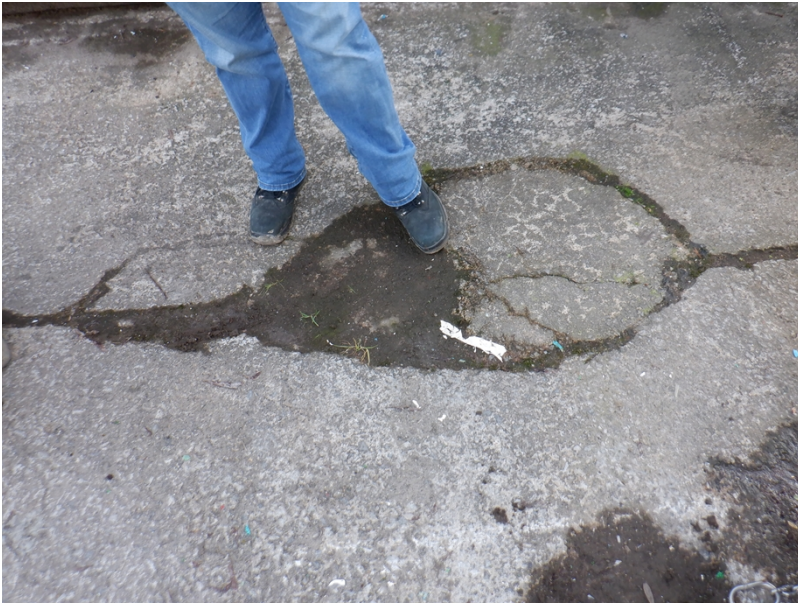
Image 2: Break in impermeable surface.
