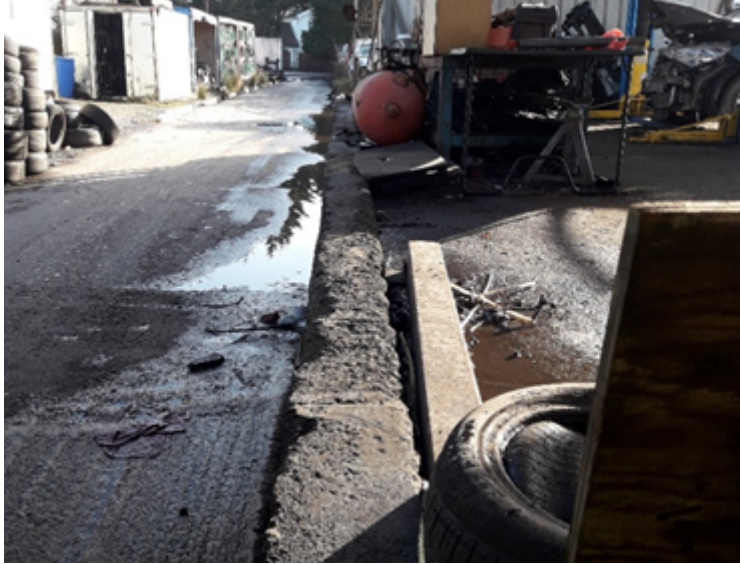
Image 2 – curbing installed in operational area
