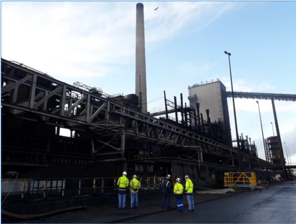
MCO coke-side looking north. Note the refurbished steel 'bridge' for the guide car running parallel to the coke oven batteries
