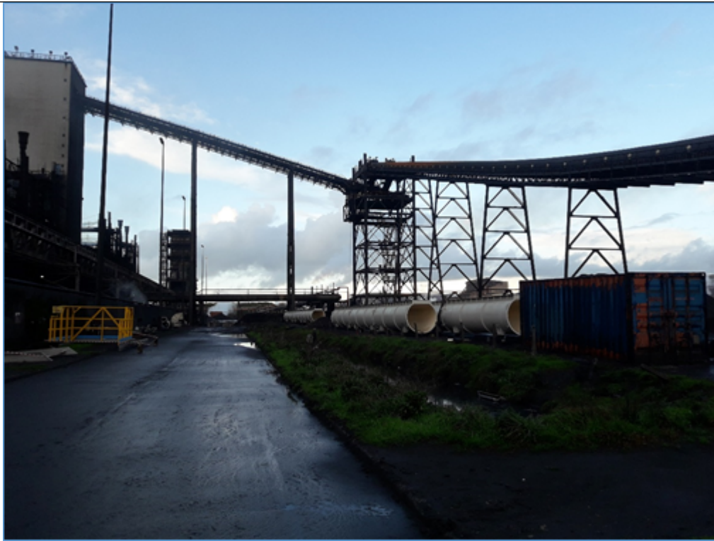
MCO coke-side looking north with new ducting components ready for installation
