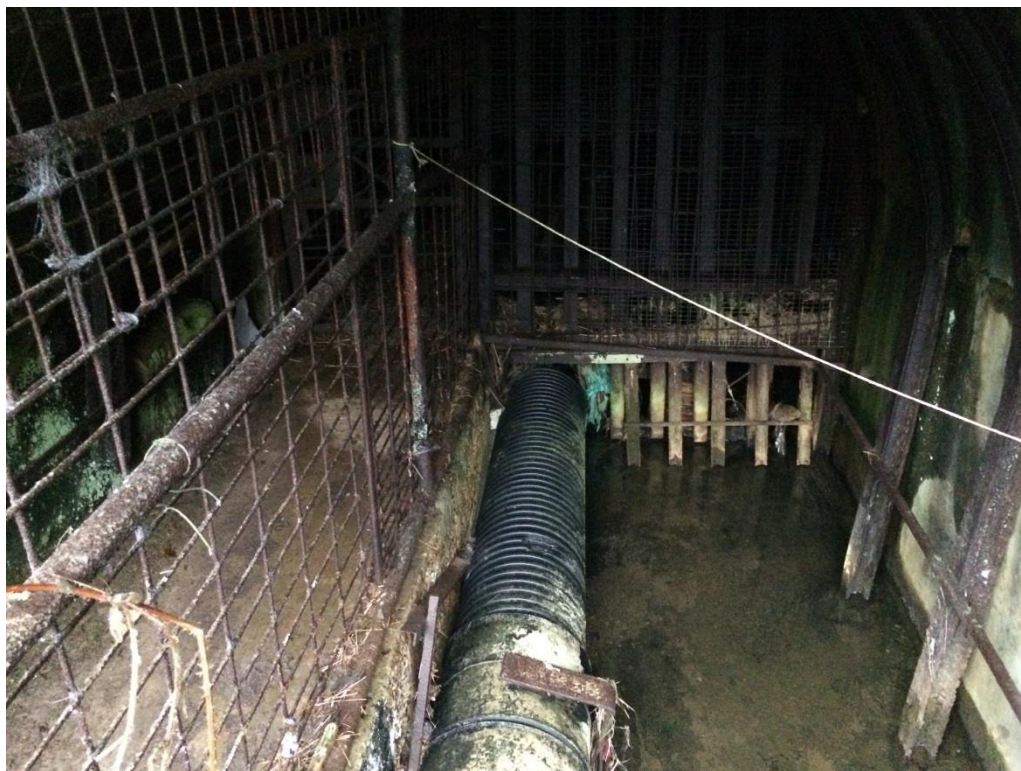
Figure B1: Photos showing the mouth of the River Arch Adit and the end section of pipework. The pipe seen in both photos is the diversion of the mine water from the adit to the mine water treatment scheme.
