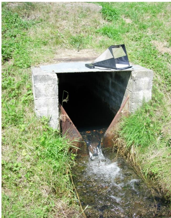
Figure B3: Photos showing two of the reed beds at the site and the now clean mine water discharging from the scheme. The lower photo shows the v-notch weir used to measure flows at the discharge point.
