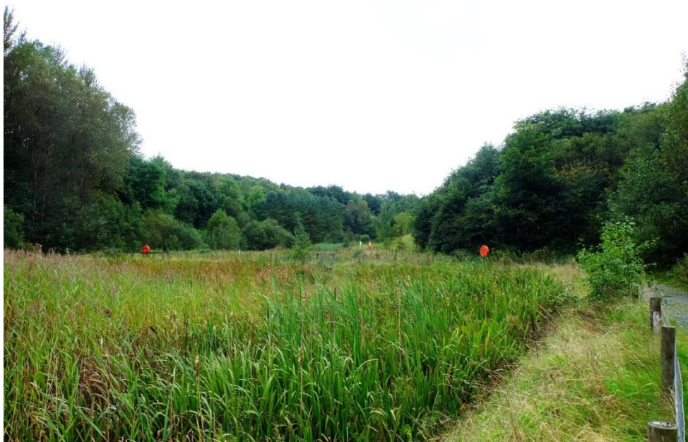
Figure B2: Photos showing the diverted ochreous mine water entering the reed bed where the oxidised iron settles from suspension.
