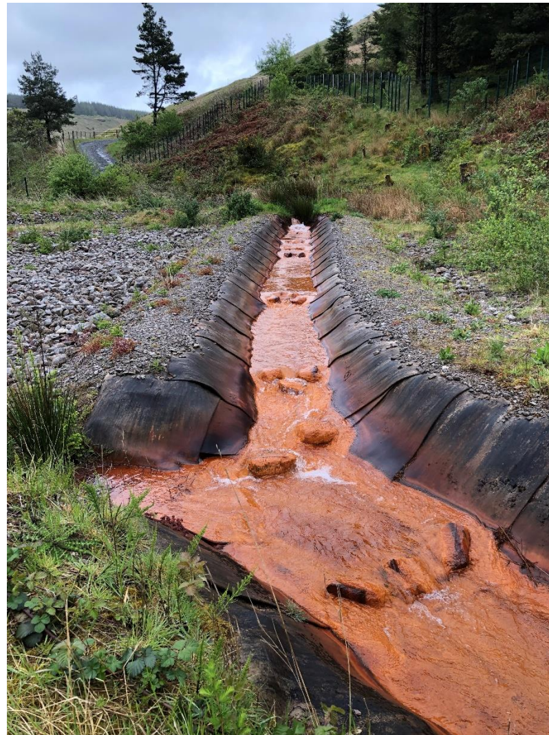
Figure B1: The left photo shows an area of mine water upwelling where the water is canalised via a concrete canvas. The right photo shows the length of the channel prior to the water entering a pipe crossing the river.
