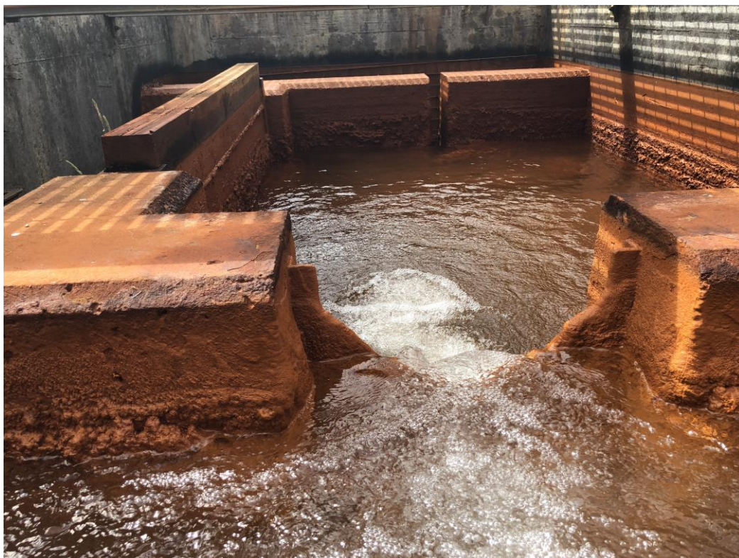
Figure B2: The left photo shows the overflow chamber with monitoring weir at the entrance to the scheme. Normal flows pass through the narrow notch (top-middle) into the treatment cells. The overflow pipe is to the left hand side below the removable weir wall (seen at the top-left). Note the ochre staining on top of the walls, and the tide mark (right wall) indicating that overflows occur. The right photo shows the engineered overflow points in the brick walls between cells.
