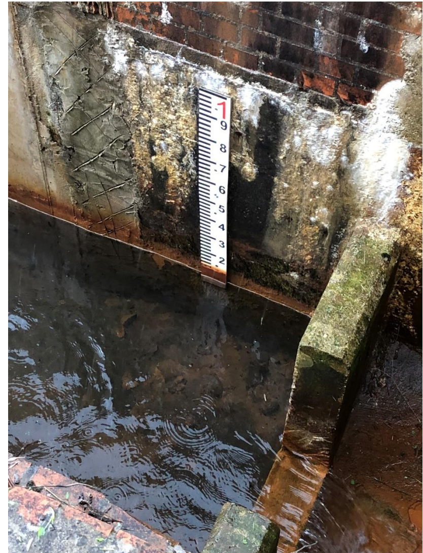
Figure B4: Both photos show the scheme discharge point where flows are measured via a gauge board and rectangular weir.
