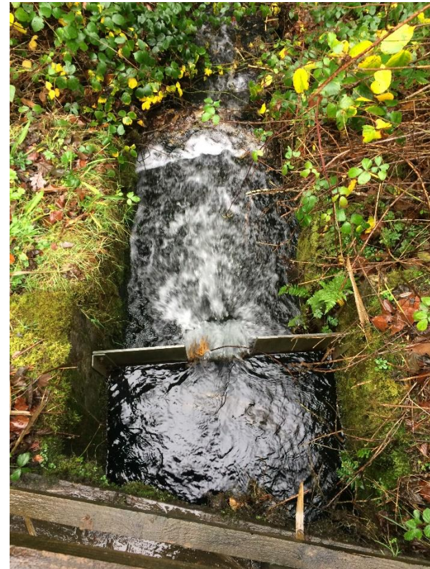
Figure B4: Photos show the now clean mine water discharging from the site. A rectangular weir allows flows to be measured at the discharge point.
