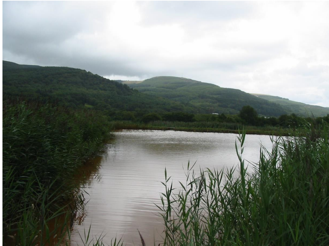
Figure B2: Photos of the two settlement lagoons where the oxidised iron settles from suspension. Left: the adit portal lies immediately to the right (out of shot) and the primary cascade is in front of the first settlement pond.
