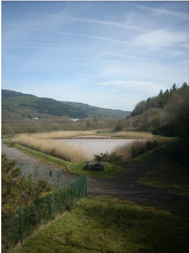
Figure B2: Photos of the two settlement lagoons where the oxidised iron settles from suspension. Left: the adit portal lies immediately to the right (out of shot) and the primary cascade is in front of the first settlement pond.
