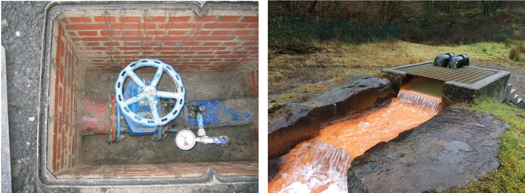
Figure B1: Photos showing the abstraction set up. Left: chamber containing one of the directionally drilled borehole pipes, with valve and pressure gauge to help control and monitor water levels within the workings. Right: two pipes delivering the mine water from the workings, by gravity, to the primary aeration cascade.
