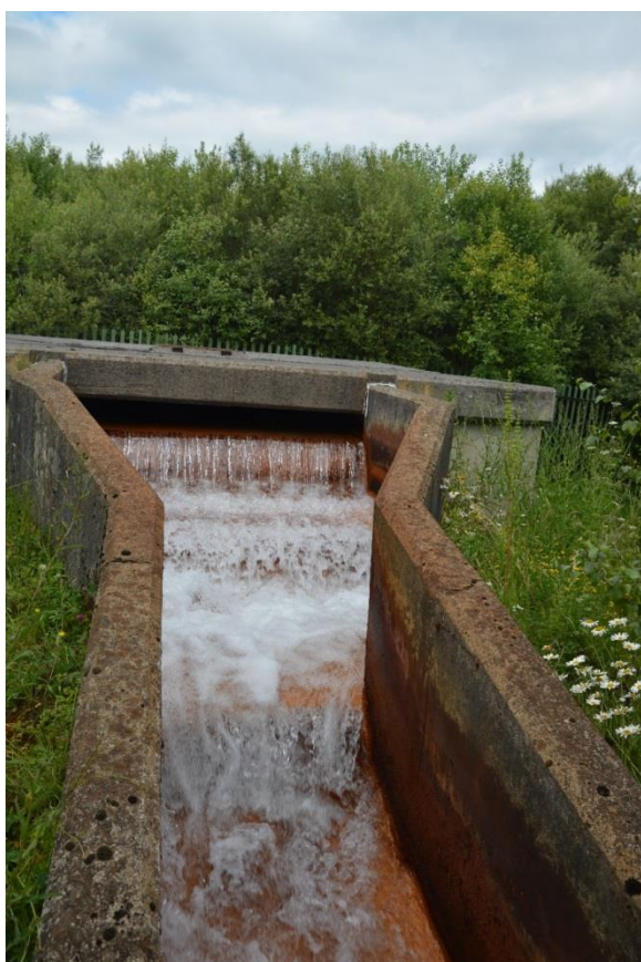
Figure B1: Photos above show the raised shaft collar (or “mine water head lifting shaft”) and cascade at the front of the structure. The raised shaft collar is designed to increase the level of the mine water to enable it to flow, by gravity, down the cascade into the settlement lagoons and thus the treatment system.
