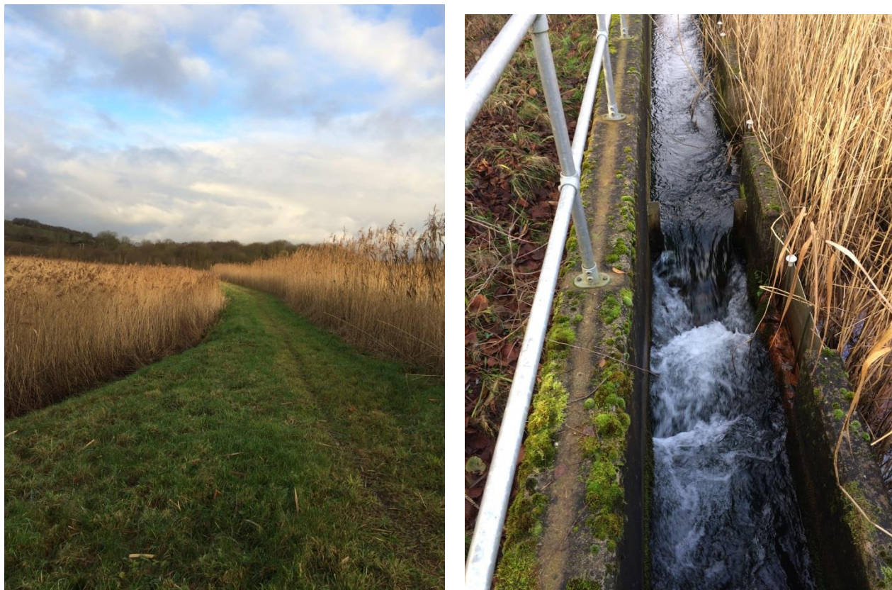
Figure B3: Photos showing two of the reed-beds at the site and the treated mine water discharging from the scheme. The right photo shows the flow monitoring weir. Both photos were taken on the 5 th December 2017.
