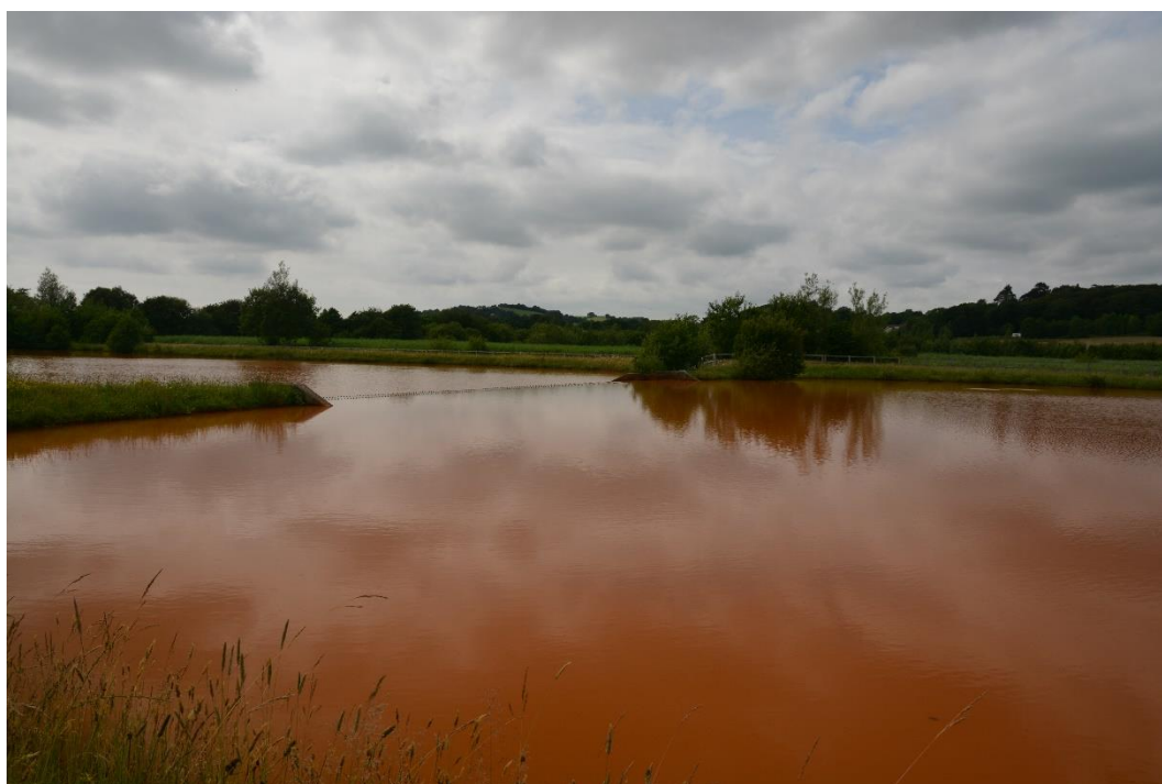
Figure B2: Photos showing water entering the settlement lagoons where the oxidised iron settles from suspension. Top photo taken 05/12/2017, lower photo taken 28/06/2017.
