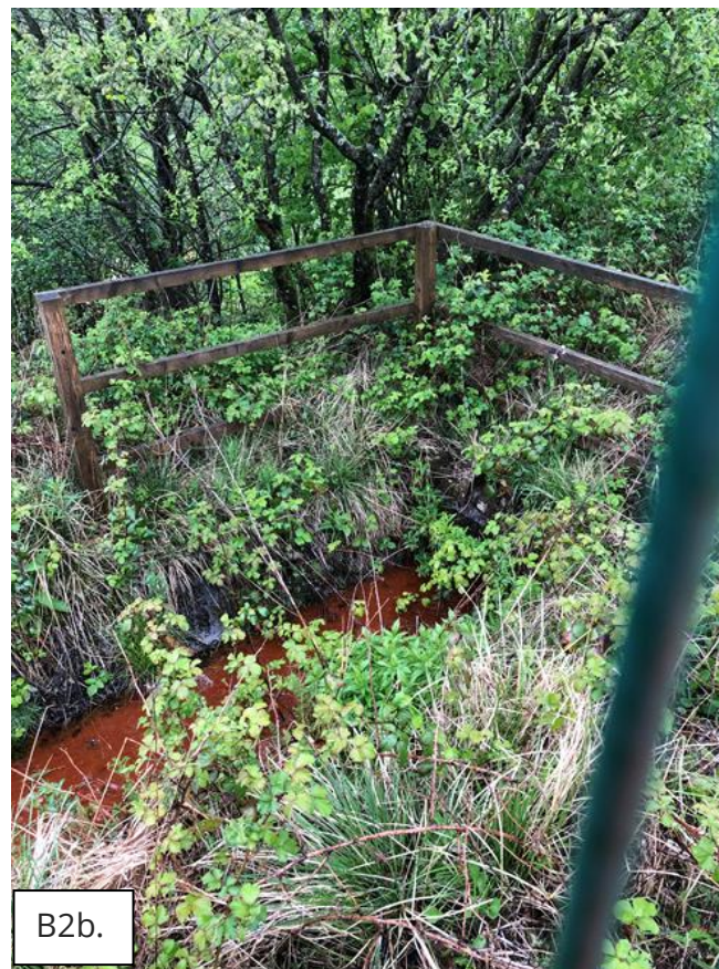
Figure B2: Photos showing the mine water emergence and capture at Whitworth B B2a: Boggy ochreous area where Whitworth-B mine water upwells, and is collected, photo taken in low flow conditions. B2b: Lined channel transporting Whitworth B mine water to the treatment scheme
