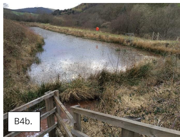
Figure B4: Photos showing Gwenffrwd/ Whitworth B scheme: B4a: Cascade (or Ochre Accretion Terrace, OAT) into the scheme B4b: Photo of settlement lagoon, cascade into scheme partially visible (located upper centre of photo). B4c: Gwenffrwd reed bed
