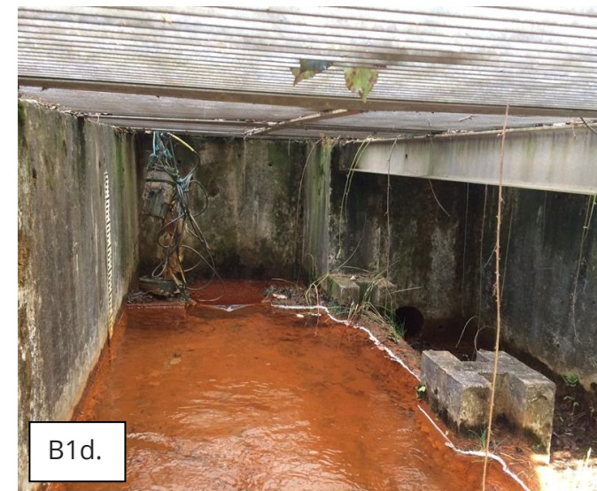
Figure B1: Photos showing the mine water emergence and capture at Gwenffrwd. B1a: Gwenffrwd mine water emerging into transfer ditch. B1b: Ditch transporting mine water towards scheme B1c: Overflow chamber collecting mine water at end of ditch B1d: Inside overflow chamber, v-notch weir for flow measurements.
