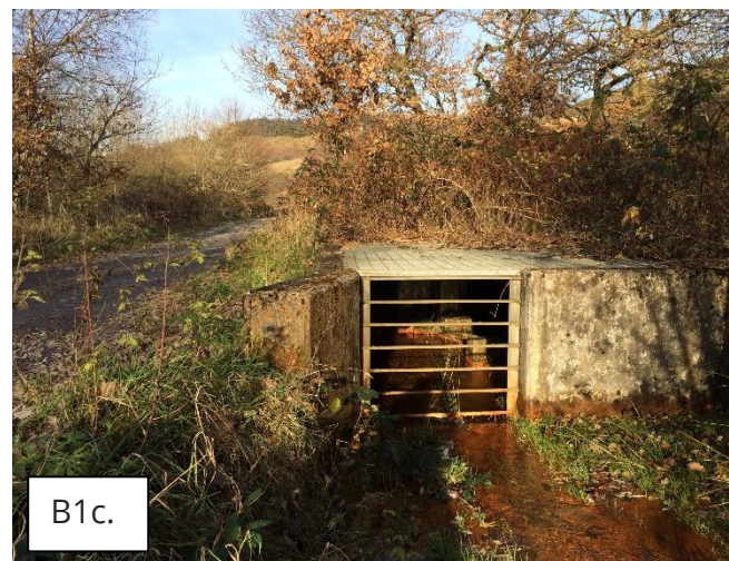
Figure B1: Photos showing the mine water emergence and capture at Gwenffrwd. B1a: Gwenffrwd mine water emerging into transfer ditch. B1b: Ditch transporting mine water towards scheme B1c: Overflow chamber collecting mine water at end of ditch B1d: Inside overflow chamber, v-notch weir for flow measurements.
