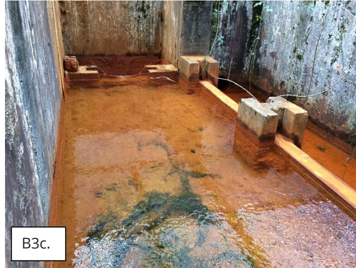
Figure B3: Photos showing the mine water emergence and capture at Whitworth A B3a: Upwelling of Whitworth A Adit mine water B3b: Overflow chamber collecting emerging mine water. B3c: Inside the Whitworth A overflow chamber – overflows occur on the right when high flows overtop the removable weir boards B3d: Whitworth A v-notch weir for flow measurements.
