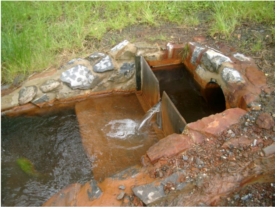
Figure B3: Photos Left – water flowing from RAPS into first settling pond. Right - showing the now clean mine water discharging from the scheme passing over the flow monitoring weir. Both photos were taken on the 5 th December 2017.
