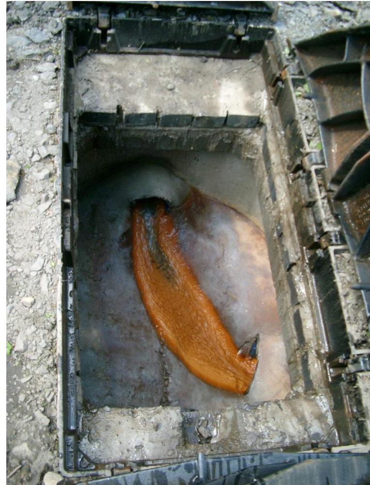
Figure B1: Photos. Left: the capture chamber looking towards the sealed adit portal; the River Cathan lies directly behind the viewpoint. Right: Looking down into the mine water capture chamber where water is diverted from its original pipeline, and to the side, towards the MWTS.
