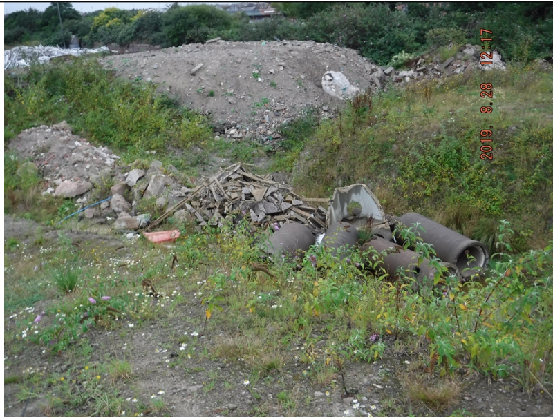
Compliant waste materials being stored on site
