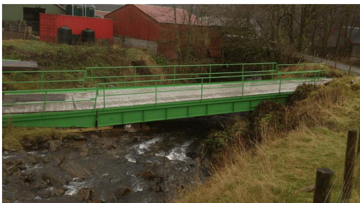
Figure 1-5 An example of a vehicular bridge
