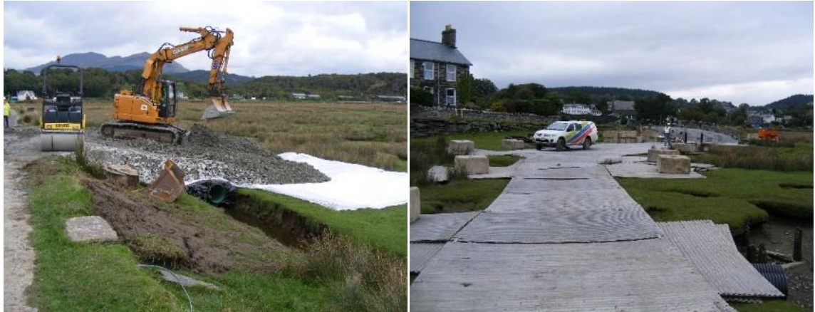
Figure 1-4 Photographs of ramp construction and trackway for previous works on Pylon 4ZC030R
