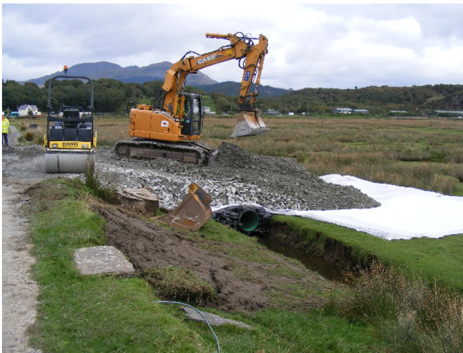
Figure 3-12 Construction of a similar culverted ramp along the existing track in 2013
