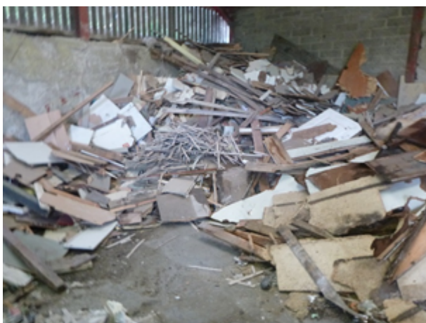
Photo 3. Drainage tank inspection hatch under waste.
