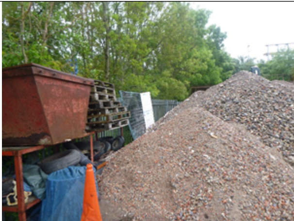
Photo 2. Crushed graded material stored on site.
