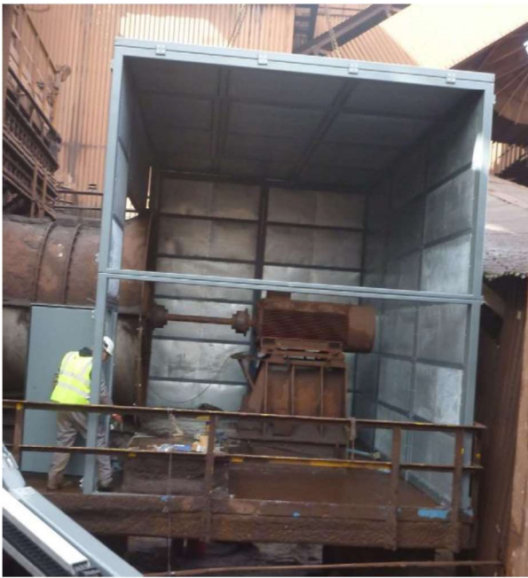
Photograph showing enclosure being fitted on the number 1 cooler fan.
