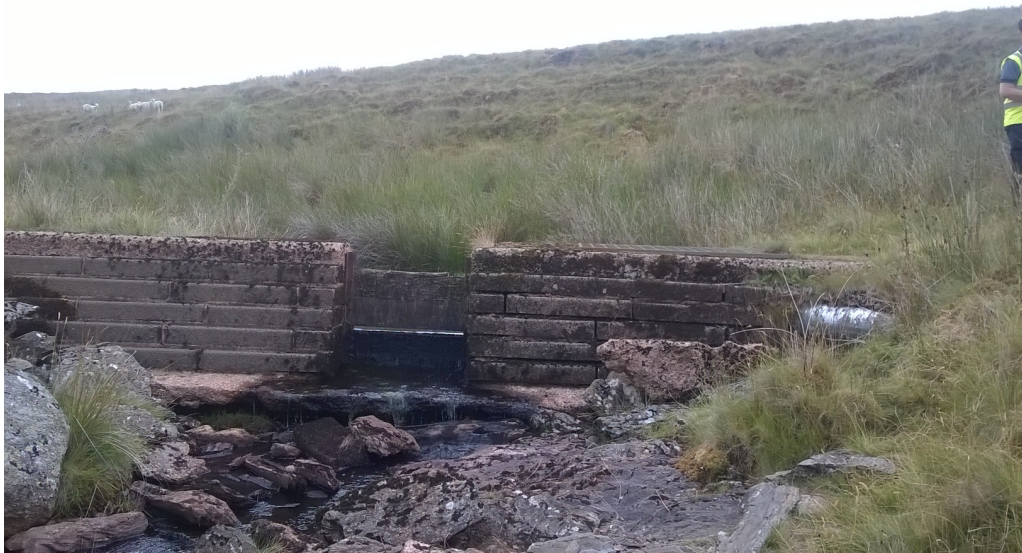
Nant y Foel Ddu Weir (intake located behind weir to right in above photo)
