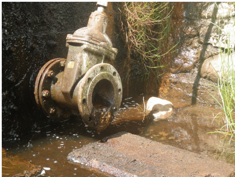
Left valve designed to deliver compensation flow
