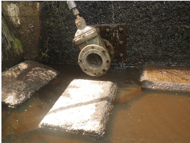
Left valve designed to deliver compensation flow
