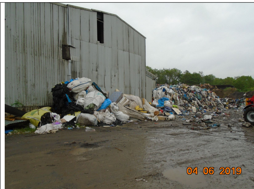
Mixed non-hazardous waste stored on permeable ground
