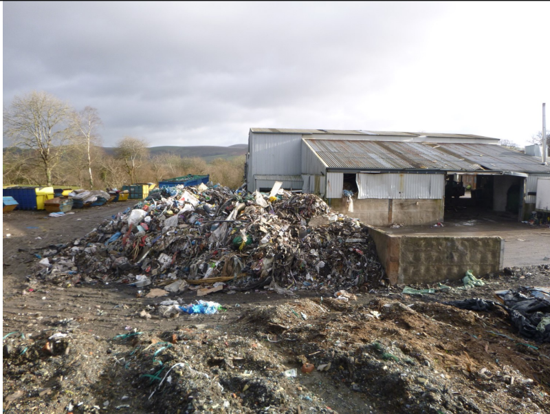
Photo showing the removal of the cardboard and the extent of the deposit of waste destined for landfill
