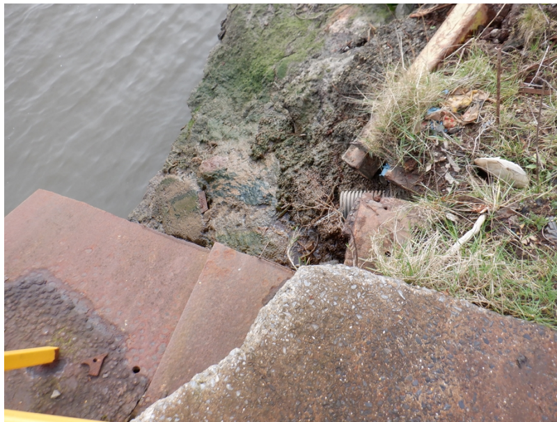
Image 3 : drainage outlet by wharf side.
