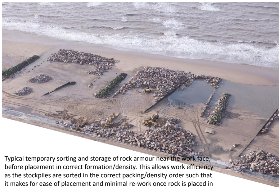
Figure 16- Typical rock armour storage near work face
