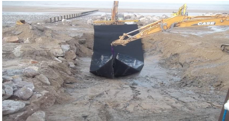
Figure 21- Typical geotextile placement
