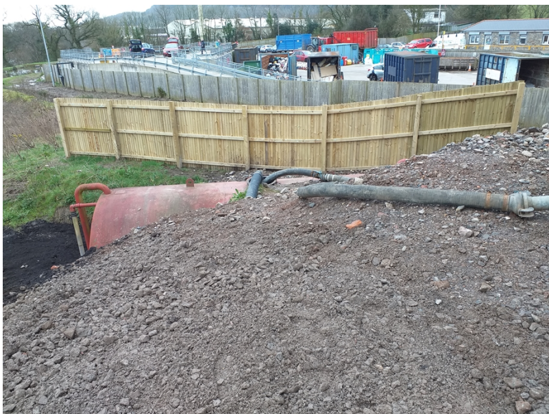
Tanker being used for site drainage
