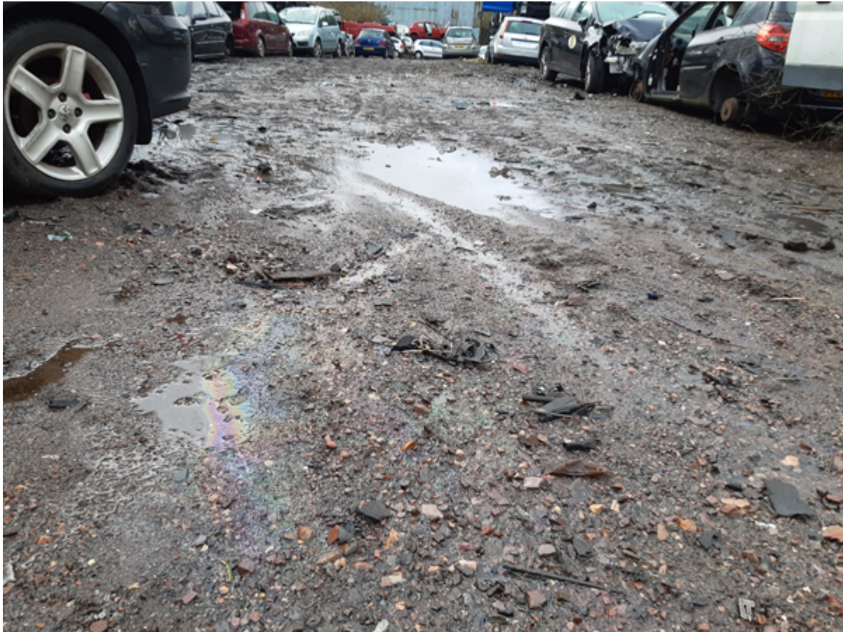
Photo: Showing oil spillage on surface of the yard.
