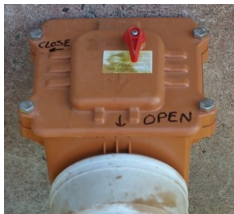
Drainage Isolation Valve
