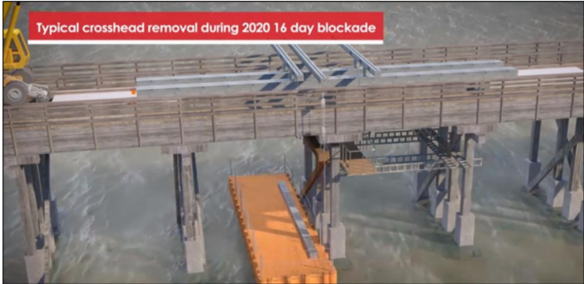
Figure 15: Cross head replacement process, supported by RRV & Barge.
