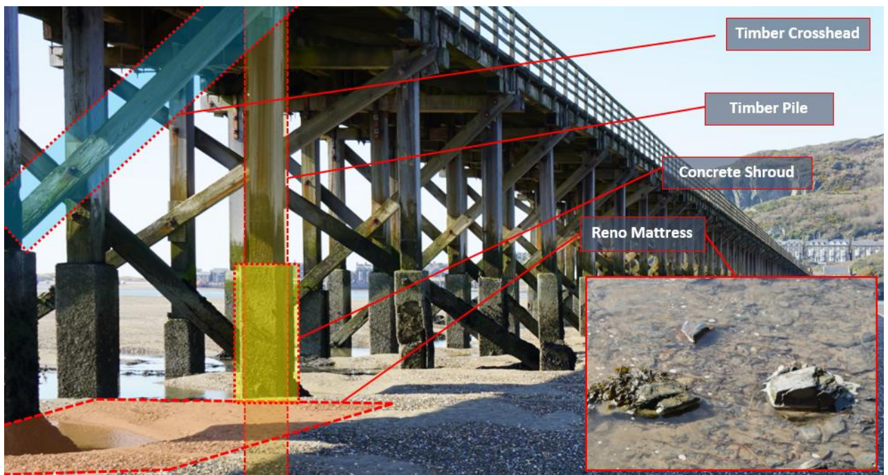
Figure 13: Illustration of individual timber structure supporting components.
