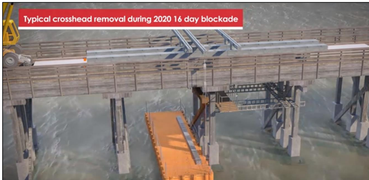
Figure 16: Cross head replacement process, supported by RRV & Barge.
