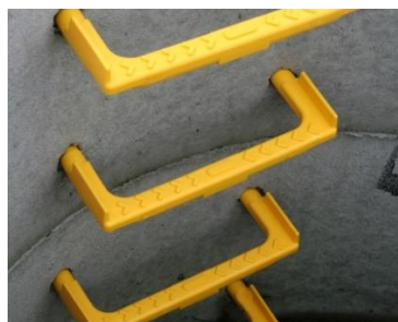
Fig 2 – Step irons with acceptable non-slip coating
