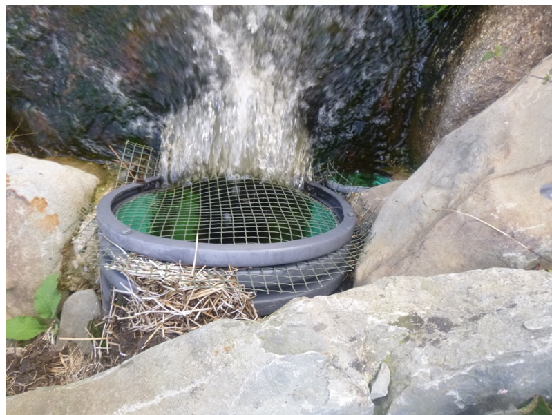
Figure 3: The outlet pipe into the Nant y Maen
