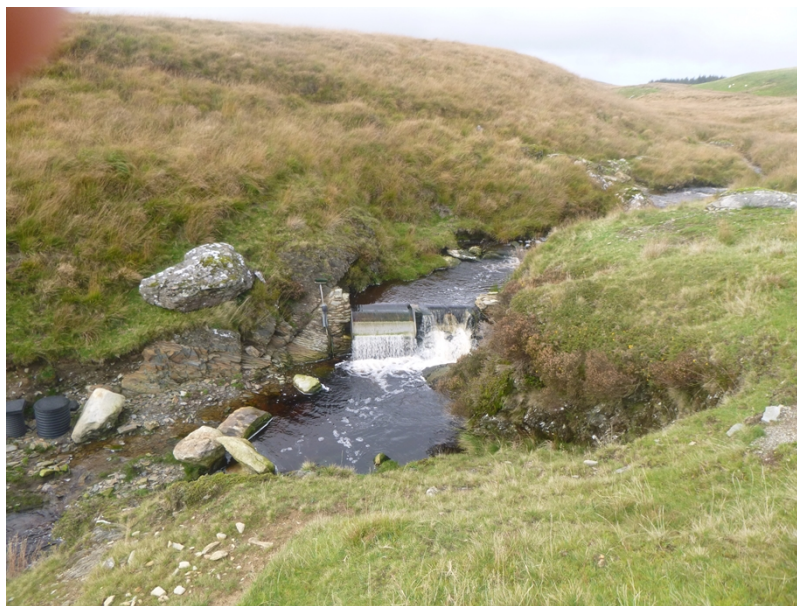
Figure 1: The intake weir on the Nant y Maen
