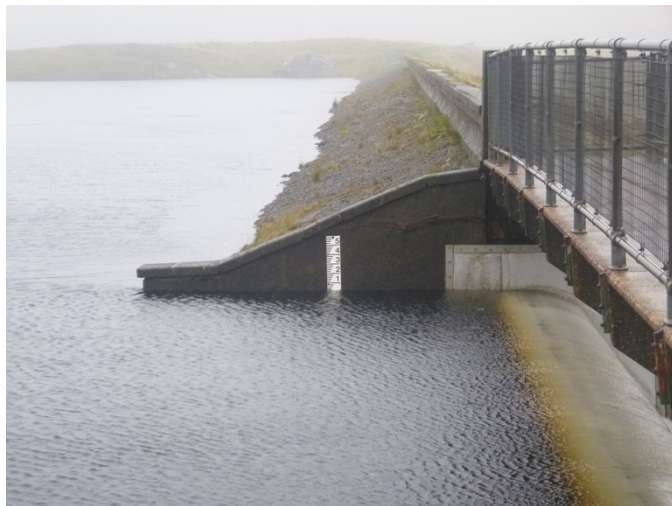
Figure 1: Llyn Teifi Top of Dam Wall
