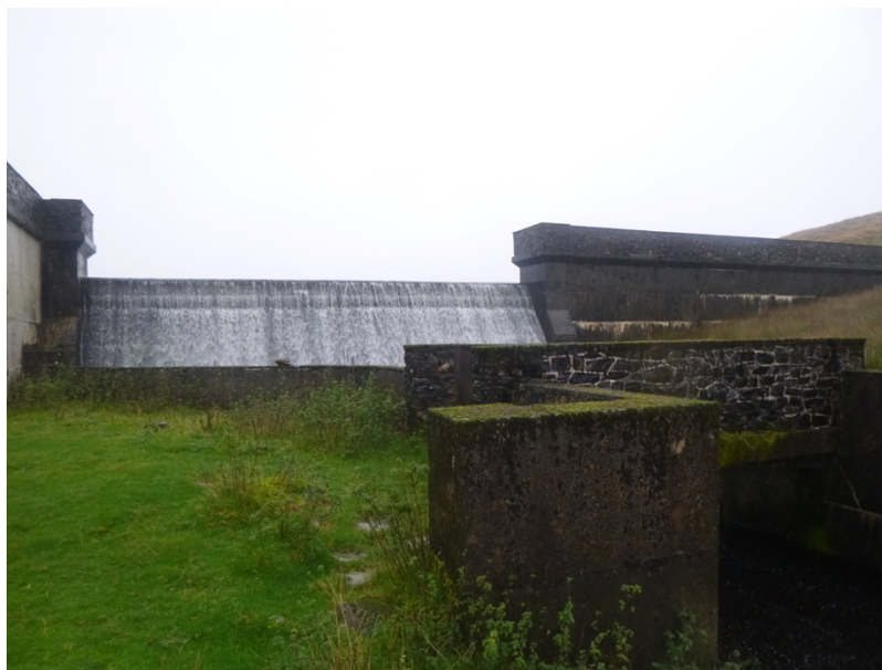
Figure 1: Llyn Egnant Dam Wall
