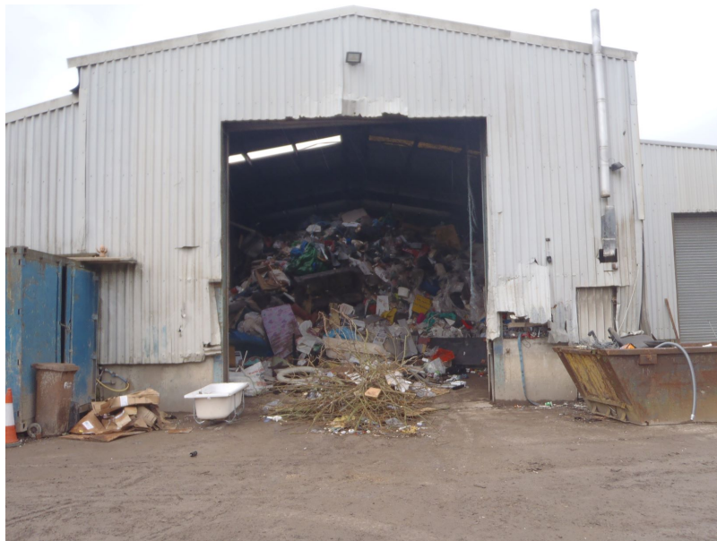
Photo of main shed with waste in the entrance
