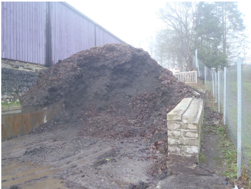
Slight over spillage of road sweepings and possible water infiltration from downpipe
