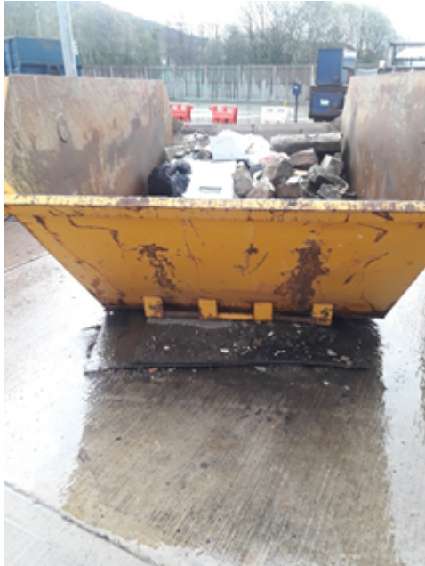
Figure 1 Rubber mats underneath skip for construction waste.
