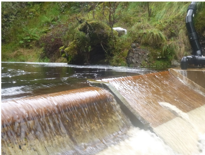
Photograph 1: Point of abstraction on 25/09/2019
