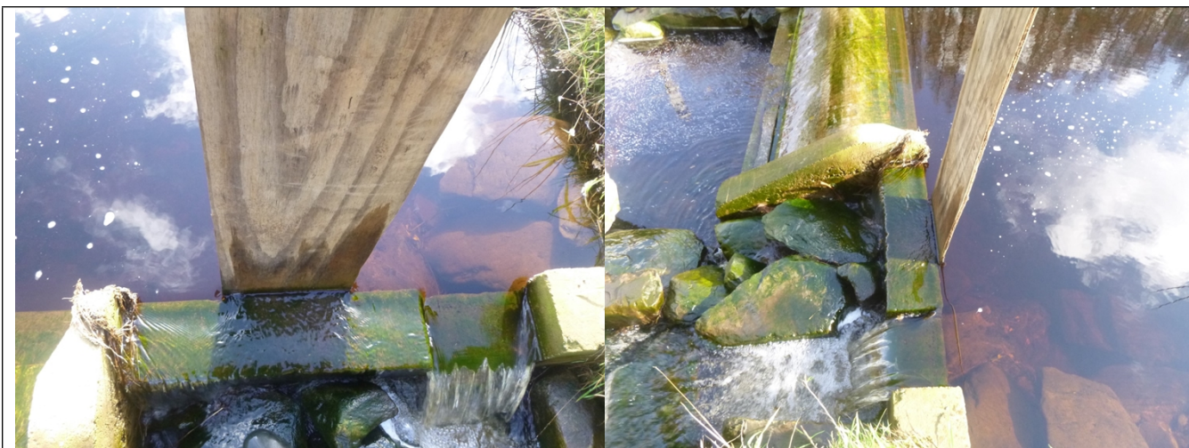
Photograph 3: Wood blocking part of fish easement
