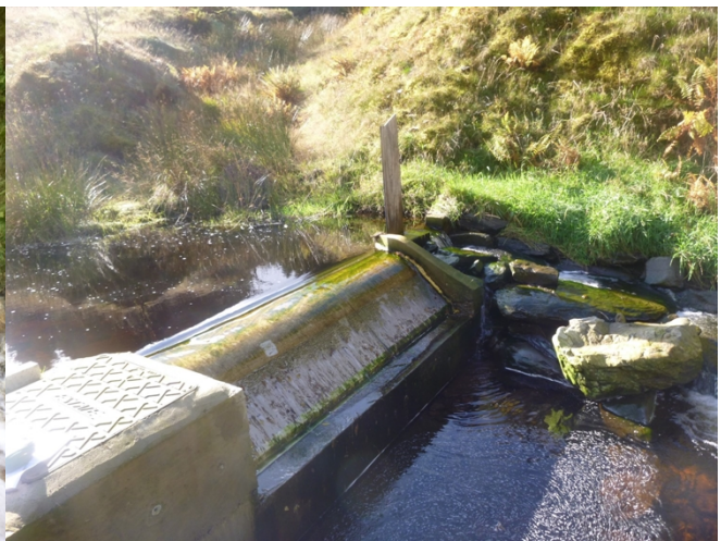
Photograph 2: Point of abstraction 23/10/2019
