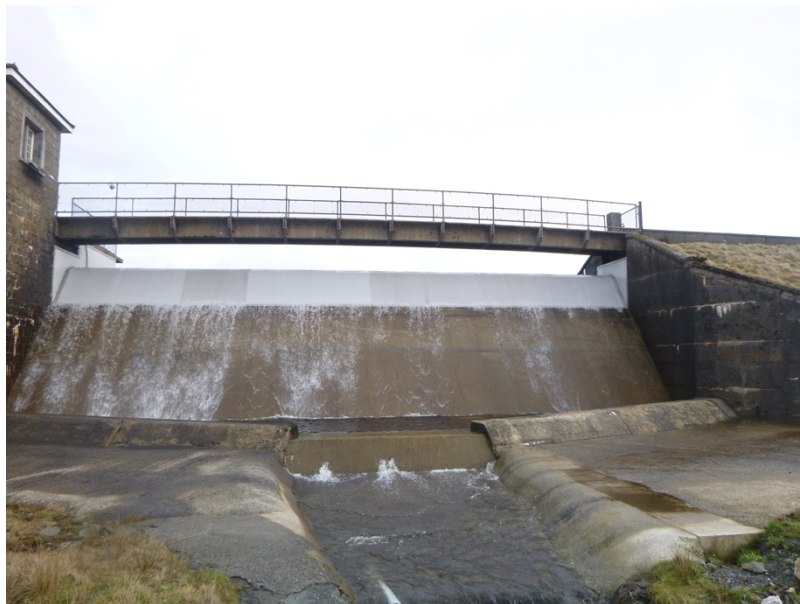
Figure 1. Llyn Teifi Dam Wall
