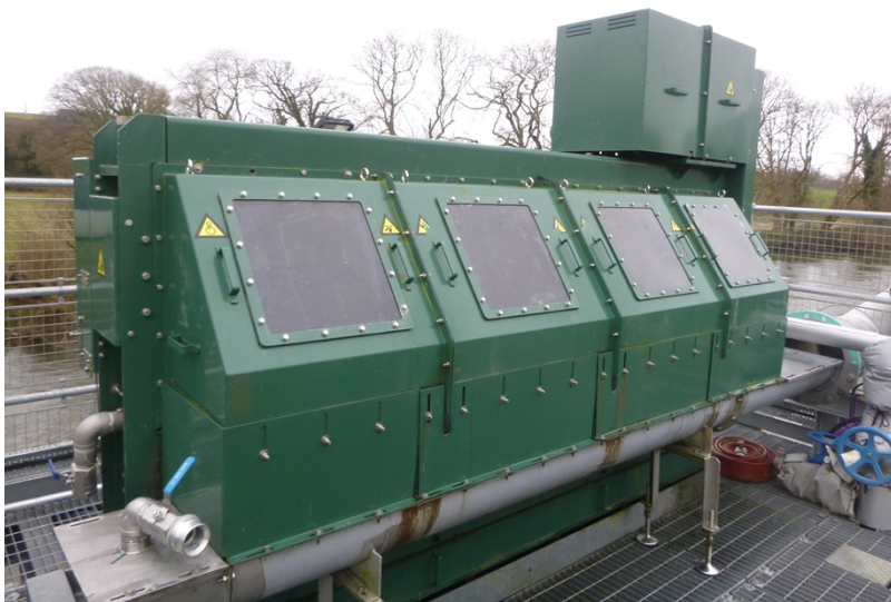
Figure 1: Screen at Llechryd Intake
