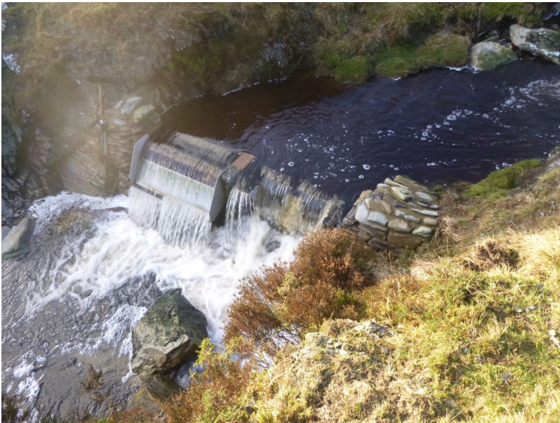
Figure 1. The intake weir on the Nant y Maen.
