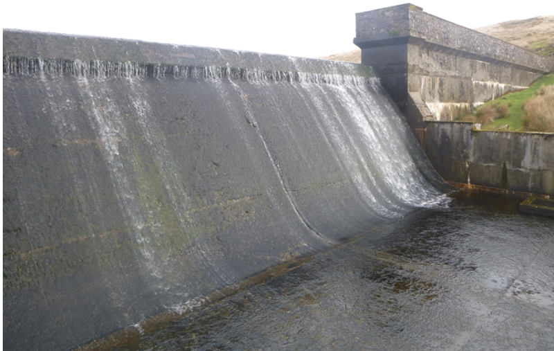
Figure 1. Llyn Egnant Dam Wall.
