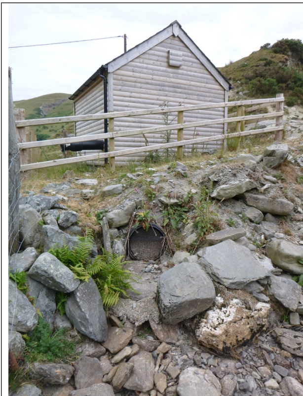
Figure 3. Discharge point into Nant Cwm-du with a screen over the outfall pipe.
