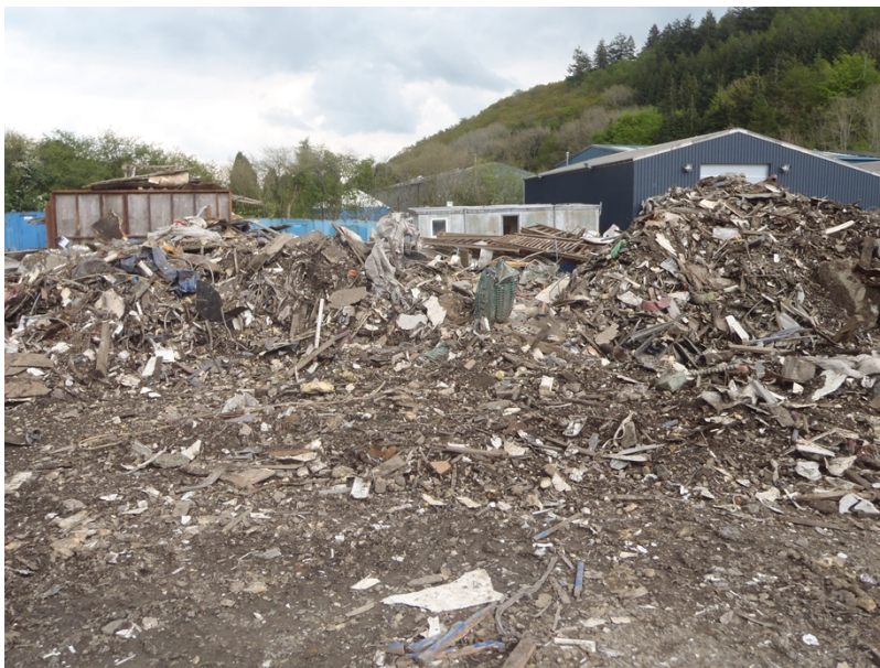
Mixed waste pile
