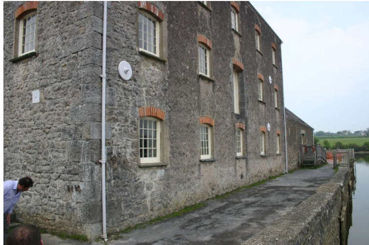
Photo 3 – View of causeway, footpath and Mill House (with disabled ramp in background)
