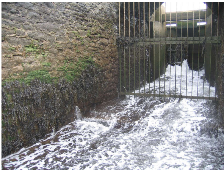
Photo 2- View of sluice channel looking upstream towards the sluice gates
