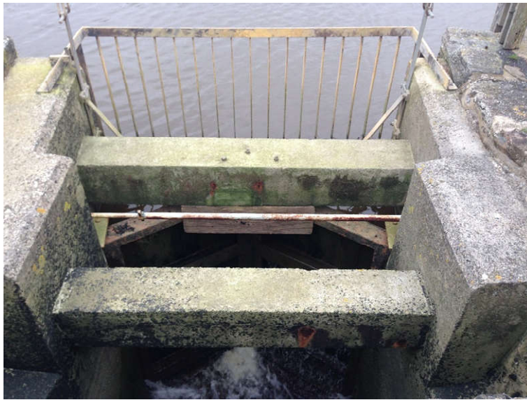
Photo 1- View of sluice gates within the sluice channel (sited below the concrete beams)
