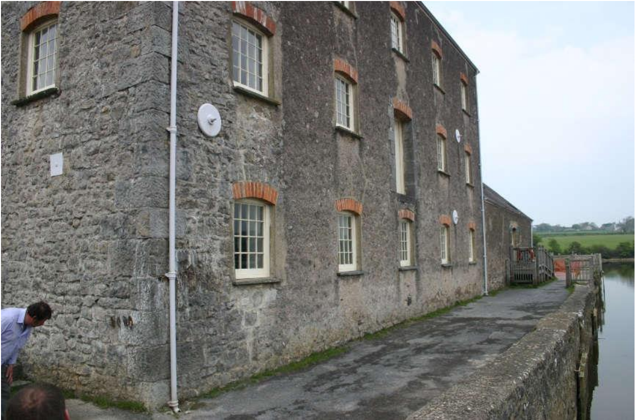
Figure 3-3 - Site access via the causeway and temporary removal of the disabled ramp (far end)
