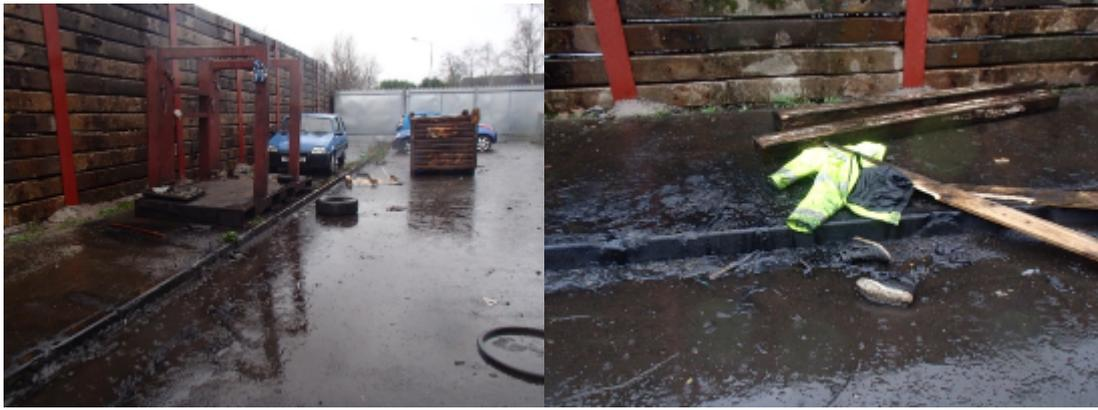
Oil was present on the road and had entered the drains alongside the kerb and from the drainage plans submitted to NRW, there are no foul drains in this area. Drainage maps held by NRW show that these drains might be connected to the surface water system.
